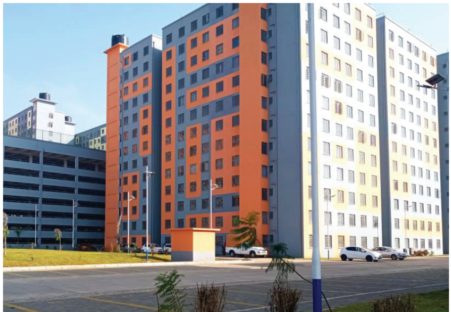
Figure 1: A case in point is the Park Road AHP, which stands as a milestone in housing delivery. Its success also underscores a broader challenge: ensuring that affordable housing remains well-managed, affordable to maintain, and sustainable in the long run .
